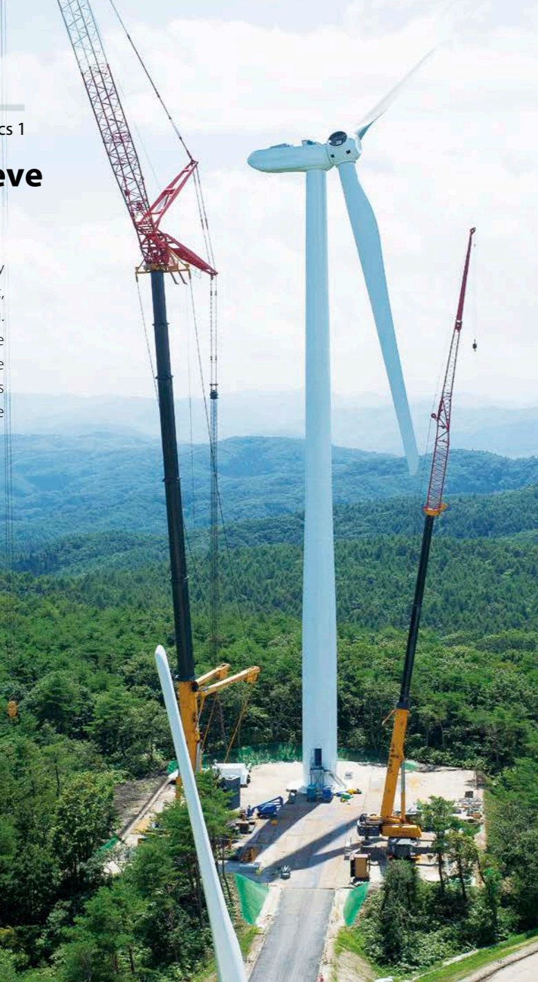
Wind power equipment installation work
